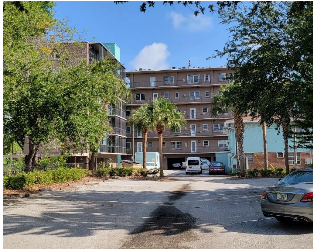
Figure 22. 750 Burlington Avenue North
