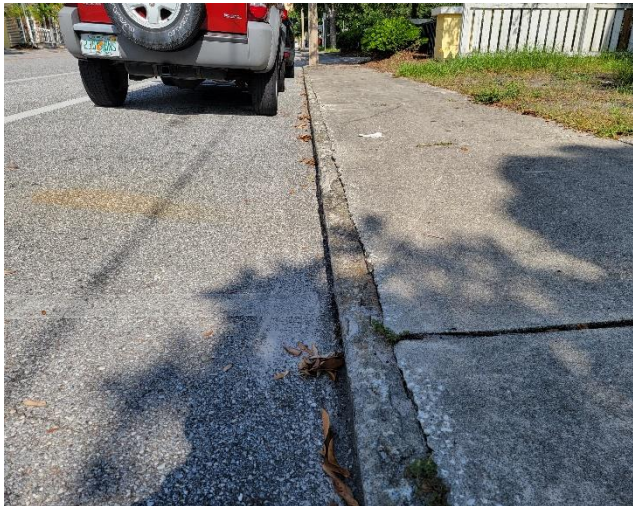
Figure 9. 2 nd Ave. No. granite curbing
